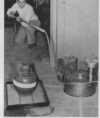
TRANSFER of radioactive isotope is made by William Dolen of the X-ray laboratory staff.
